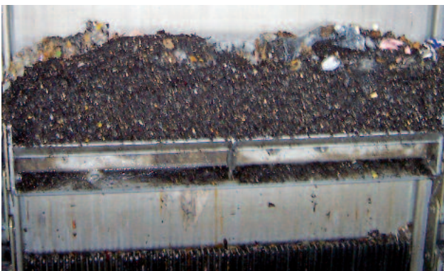
Screens with small bar spacings (here 6 mm) have specially shaped bars (tear drop design). The pressure loss is thus significantly reduced compared to flat or trapezoidal bars. The special bar shape prevents jamming of solids in the bar spacings. The screen proves thus its insensitivity to grit and gravel.
